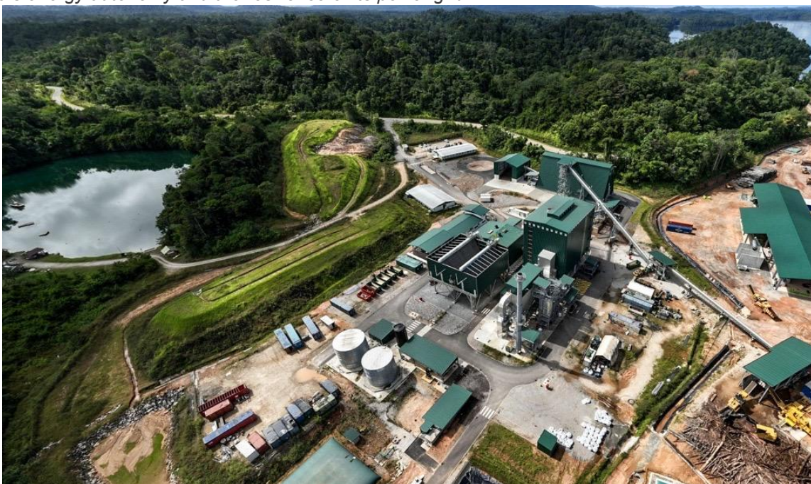
Sinnamary biomass power plant, Voltalia - Credit: SENTINEL
